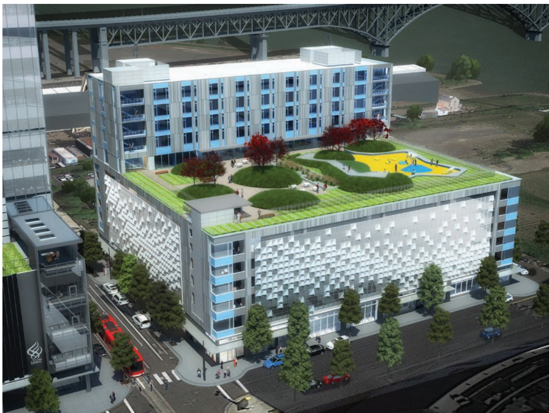
Planned new OHSU parking structure and patient housing, as seen from high over southwest corner of Bond Avenue and Curry Street. Whimsical design is said to represent flight of birds.
