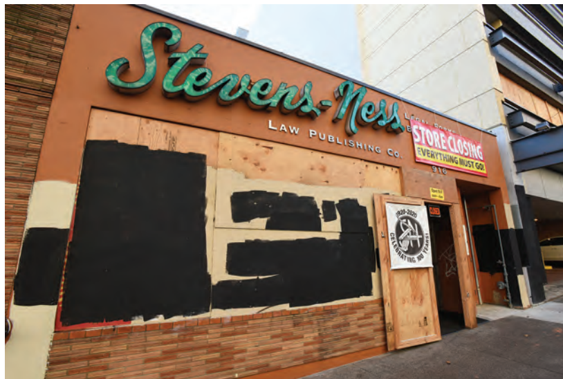
Protest-damaged Stevens-Ness, a 100-year-old company, sold legal and business forms. It shuttered its walk-in store in 2020. Photo by Robert French.
