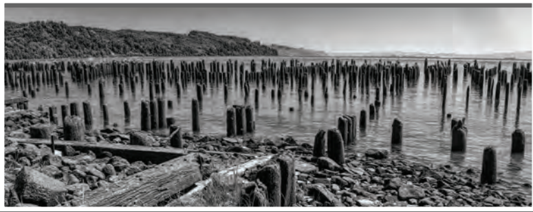
Old wood pilings, Columbia River, Washington State
