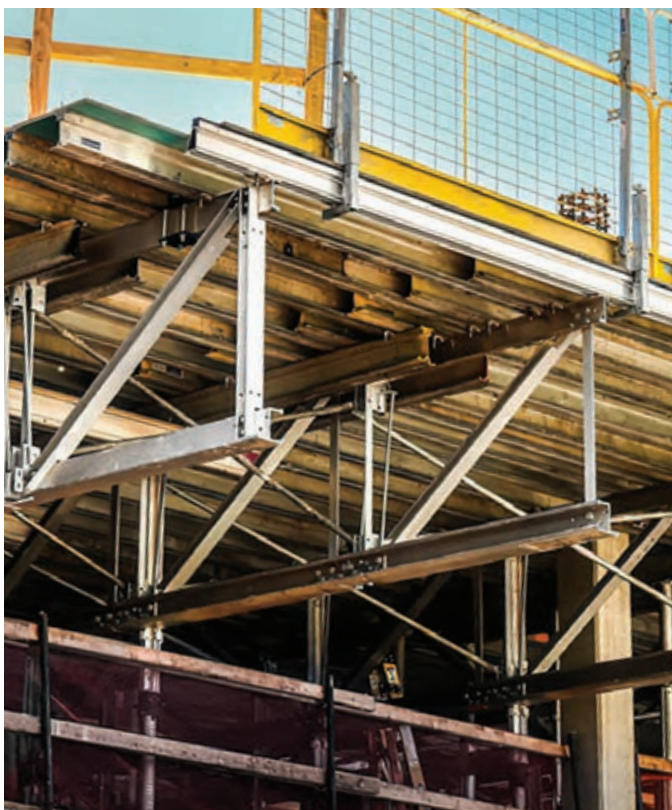
Flying trusses in Block 41.
