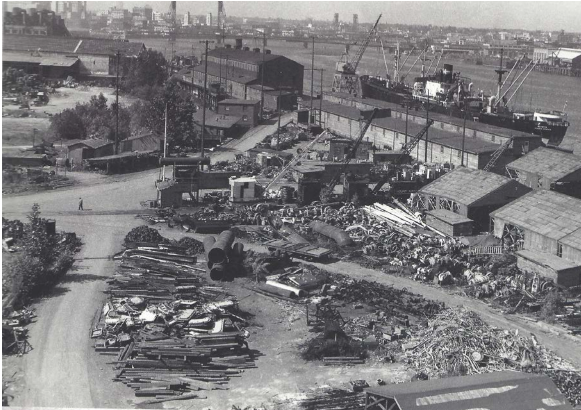
Zidell site in ship-stripping days. Photo courtesy of the Zidell Companies.
