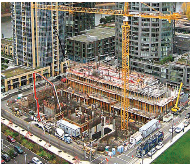
Terrace building rises as work starts on Mirabella Terrace
