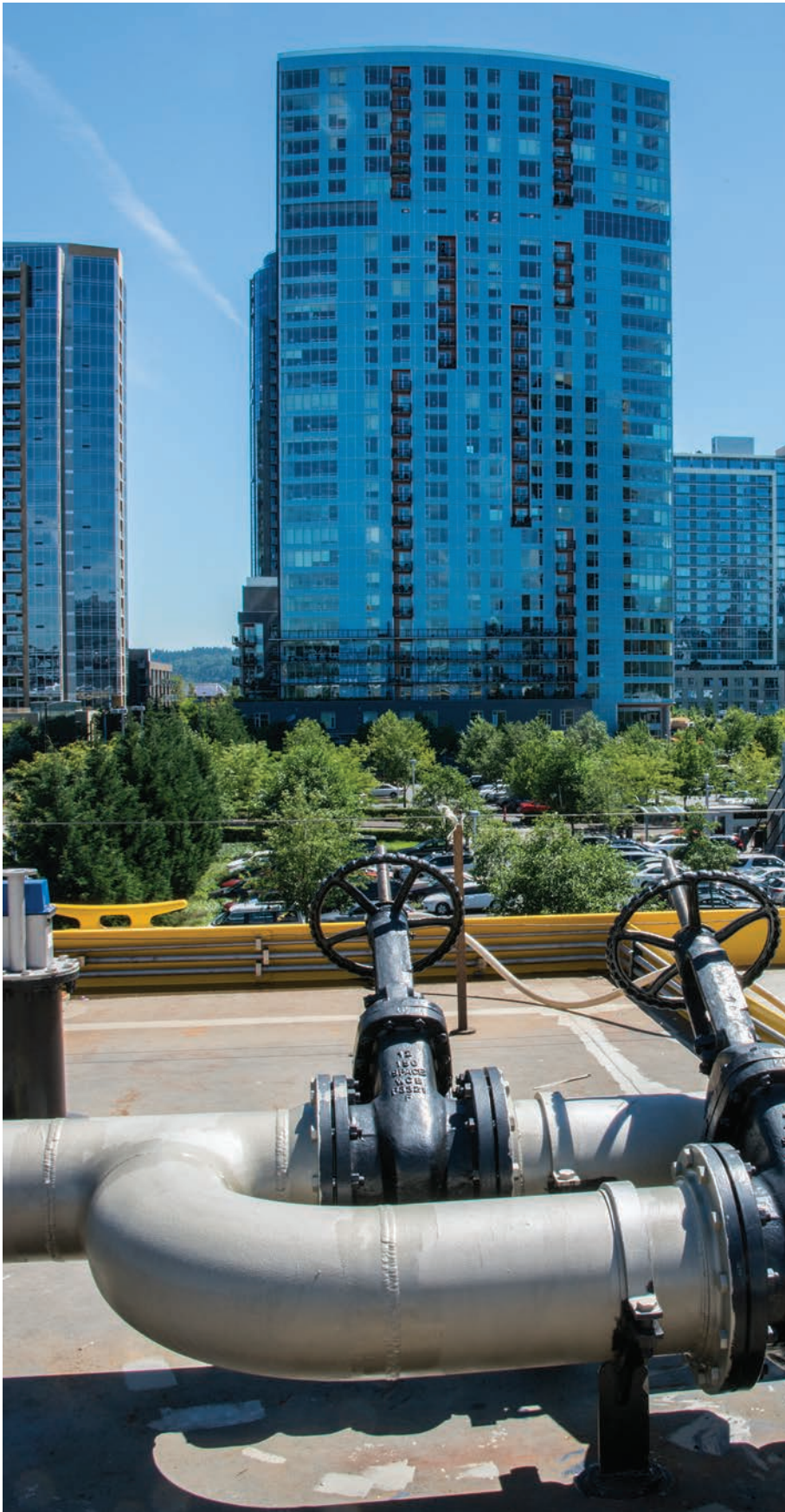
From atop Zidell's latest barge, it's easy to see why Mirabella residents keep such an eye on on all phases of barge construction.
