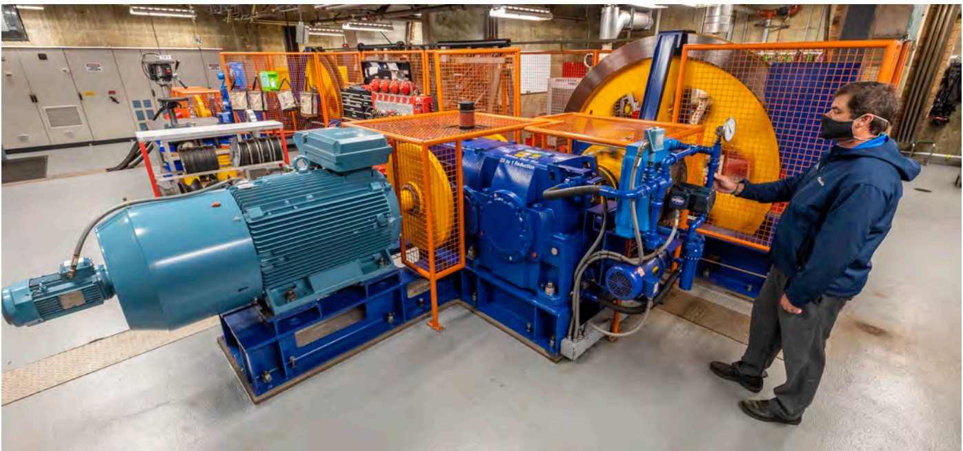
Tram general manager Ray Gardner shows visitors one of the motors that drive the bull wheel. Photo by Robert French.
