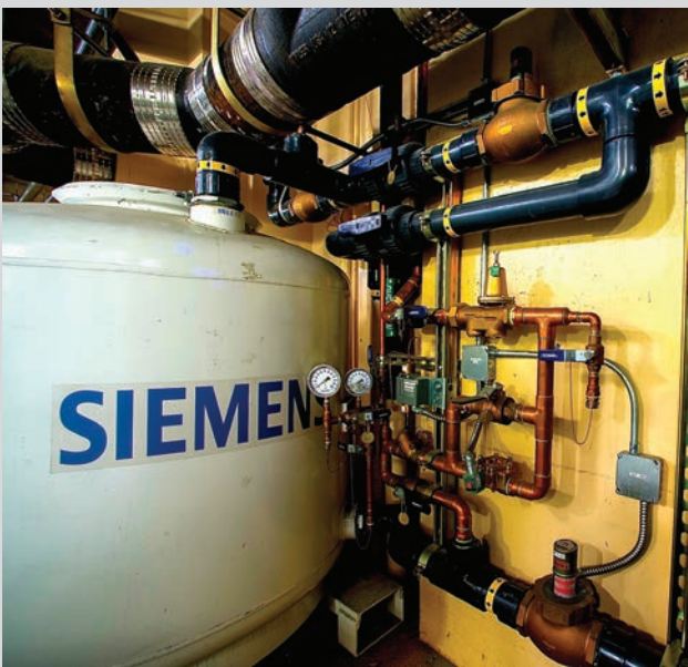
Water Recovery System – roof rainwater is captured and recycled.
